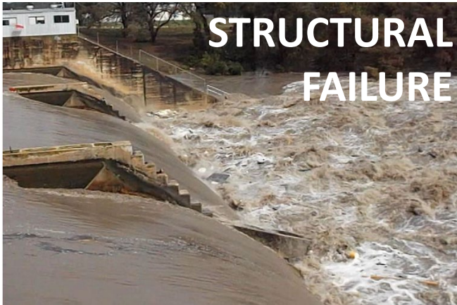
2019 Lake Dunlap Spillway Failure. Guadalupe-Blanco River Authority
